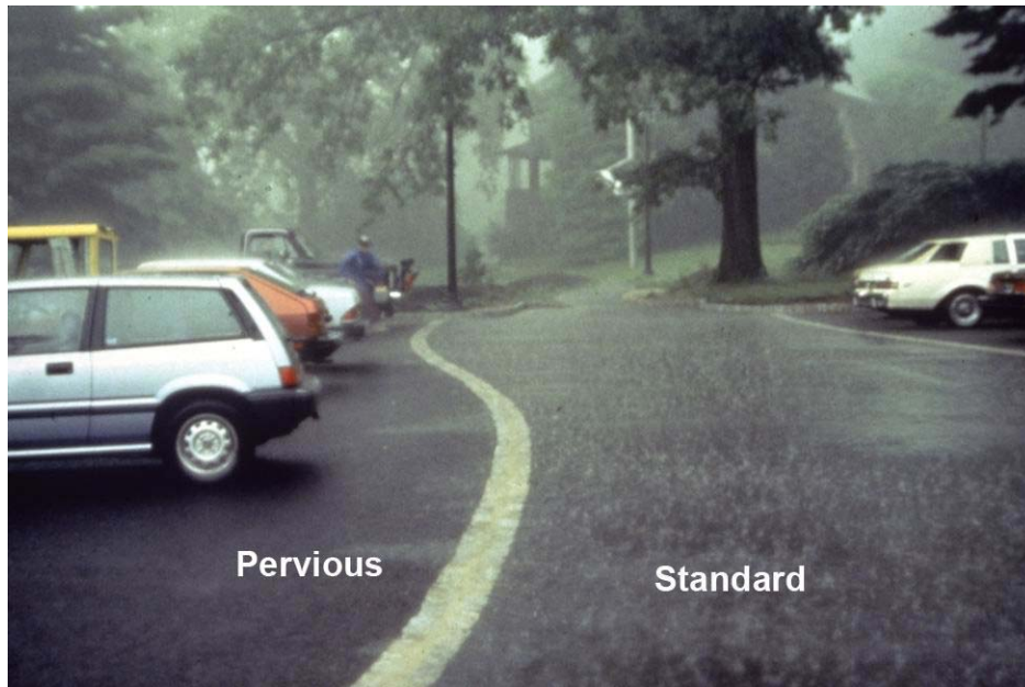
Figure 1: Routine and adequate maintenance has allowed the porous asphalt parking lot at the Morris Arboretum to still be effective 20 years after installation.
