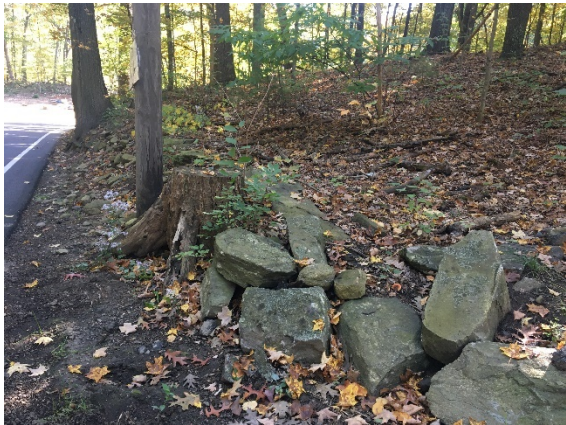
Photo 1. Stone wall along South Bolton Road.
