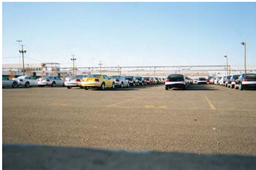
Figures 4 and 5: Neither the porous asphalt parking lot at the University of Rhode Island nor the one at the Ford Rouge Plant in Dearborn, Michigan have experienced significant snow accumulations on the pavement after multiple harsh winters.
