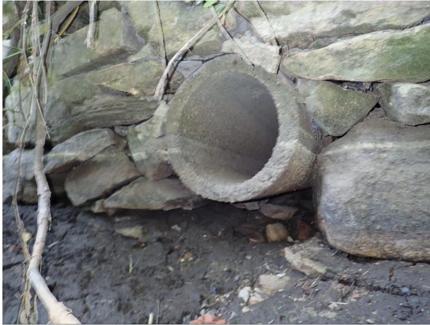
Photo 12: Undermining at Drainage Outfall
