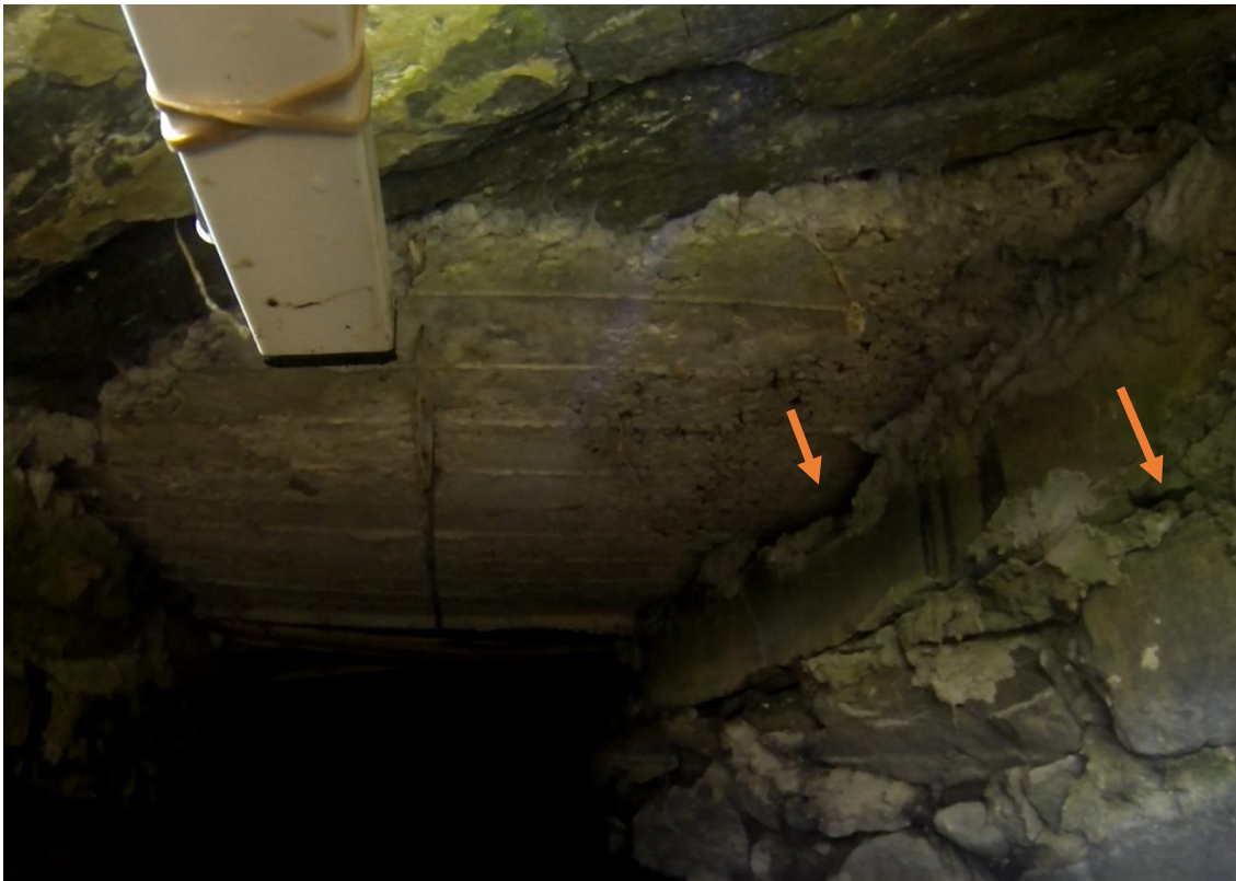
Photo 6: Voids in Culvert Walls (GoPro stillframe image)
