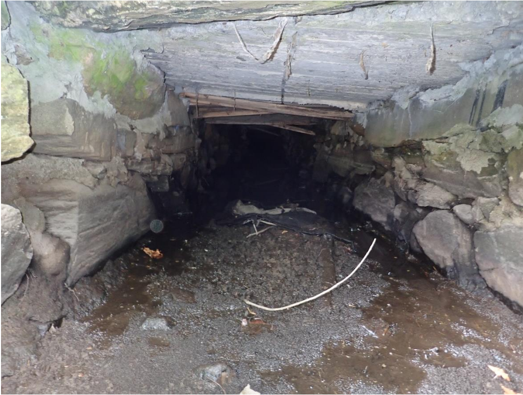
Photo 5: Culvert Outlet Interior
