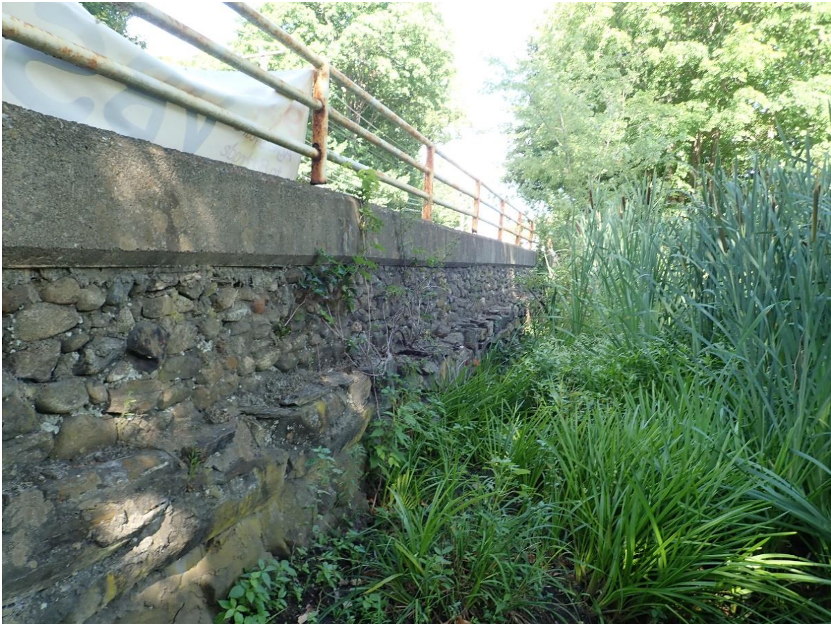
Photo 9: Downstream Retaining Wall supporting Main Street
