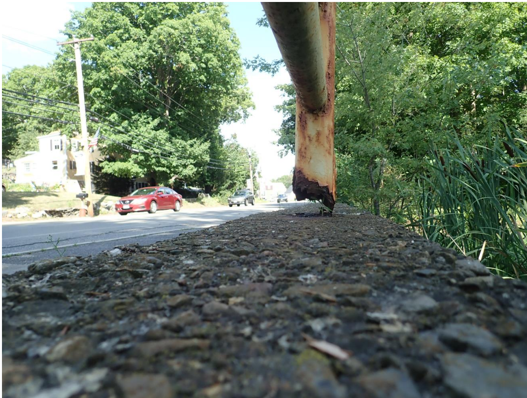
Photo 13: Guardrail Post with 100% Section Loss
