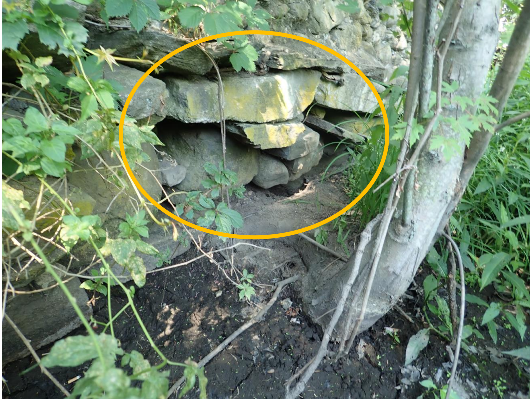
Photo 10: Dislodged Stones and Voids in Retaining Wall
