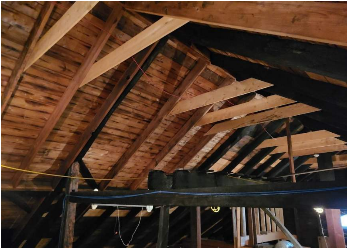
Photo S2: Rebuilt roof rafter and decking after fire.
