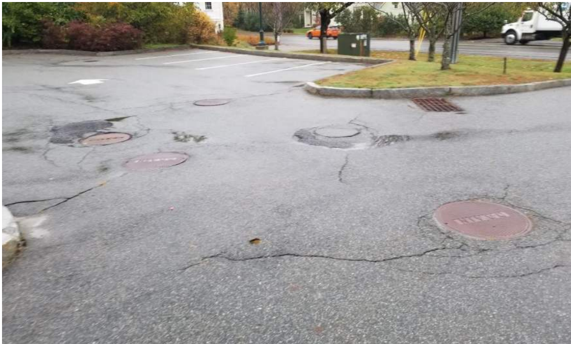
Photo C2: Bituminous concrete settling around manhole covers throughout driveway.
