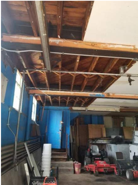
Photo S3: Cable bracing in first floor of Old Fire Station.
