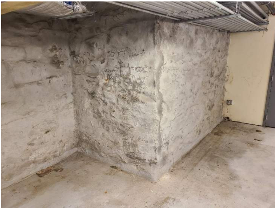
Photo S2: Foundation moisture in basement of original library should be monitored.
