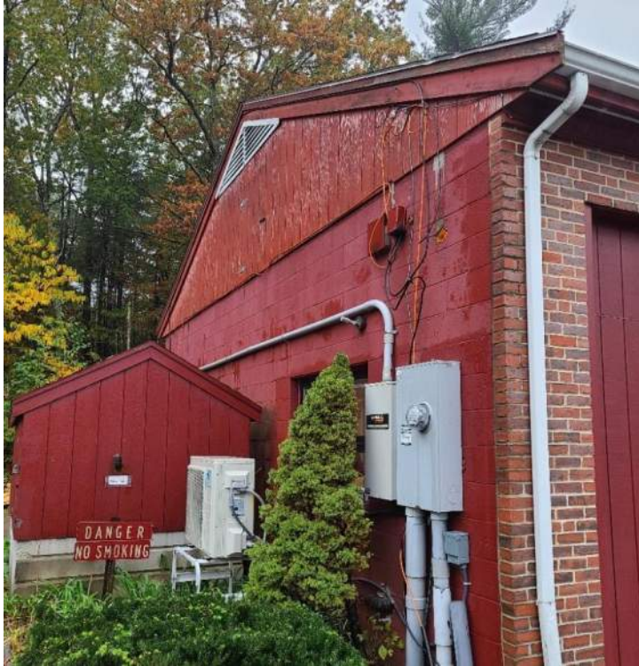
Photo S1: Exterior Paint Peeling on Garage. Typical of Admin Building too.
