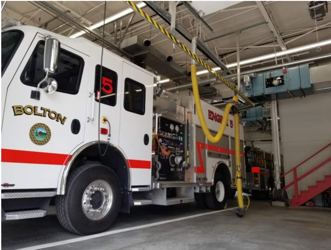
Photo H1: Gas detection for NO 2 and CO is needed in garage. Upgrade ventilation controls based on gas level.
