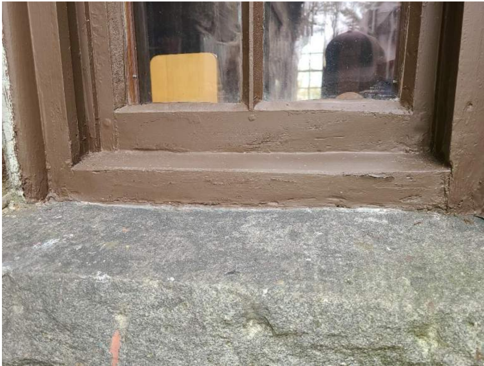
Photo S3: Rot on sills of small double hung windows. Sill rot throughout building.
