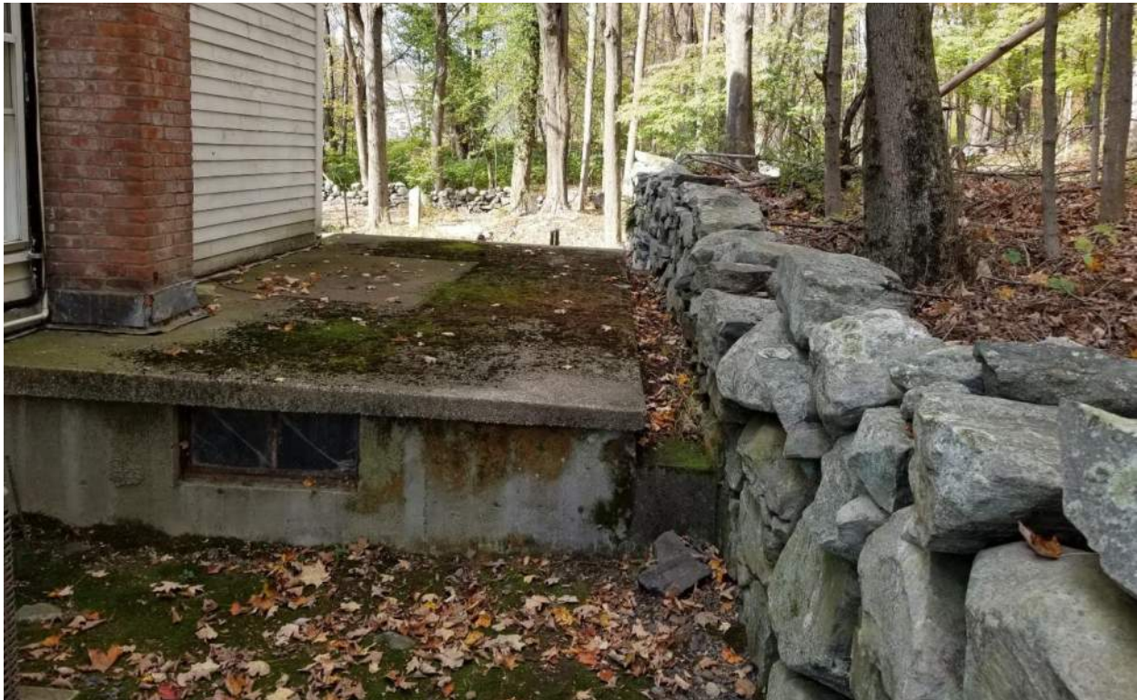
Photo C1: View of boiler room and stone wall behind building. Water weeps into building at this point. Investigate installation of either a drainage system installed behind wall to direct flow around building or an interior or exterior cutoff drain below boiler room floor elevation.
