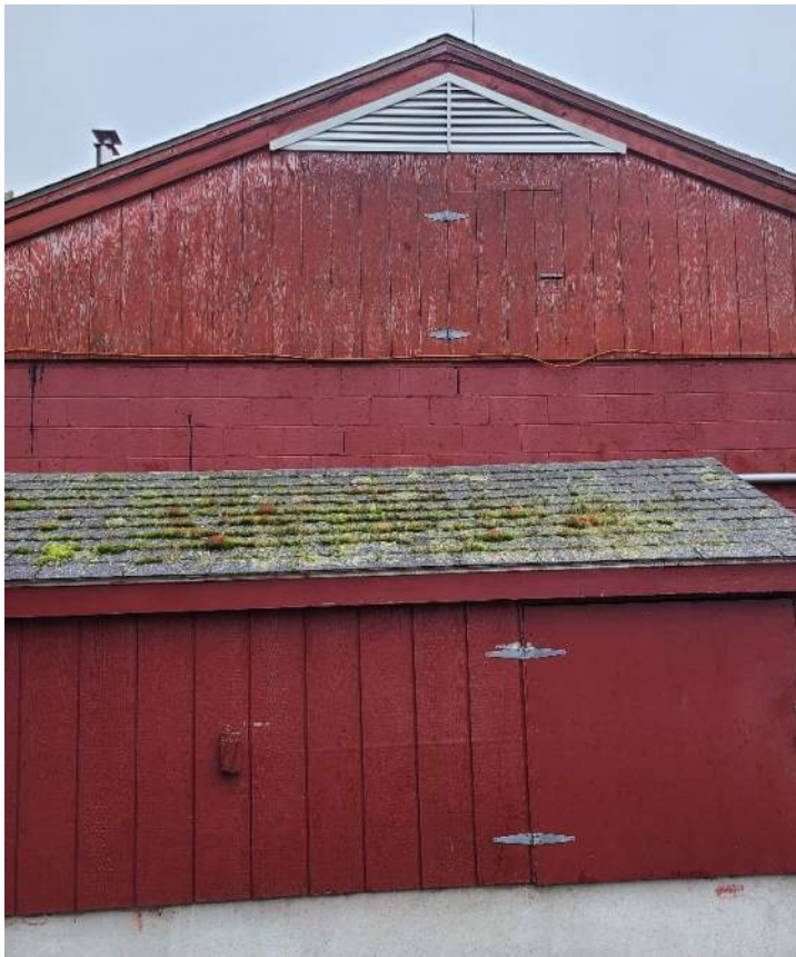
Photo S2: Oil tank shelter shingles covered in moss.
