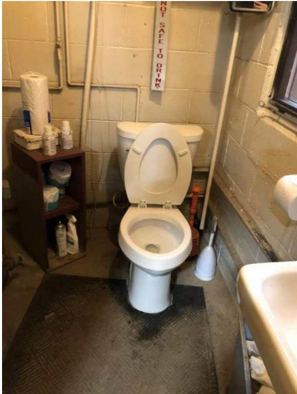
Photo P1: Garage bathroom needs exhaust fan. No showers for employees and no female-specific bathroom. Replace cesspool with tight tank.
