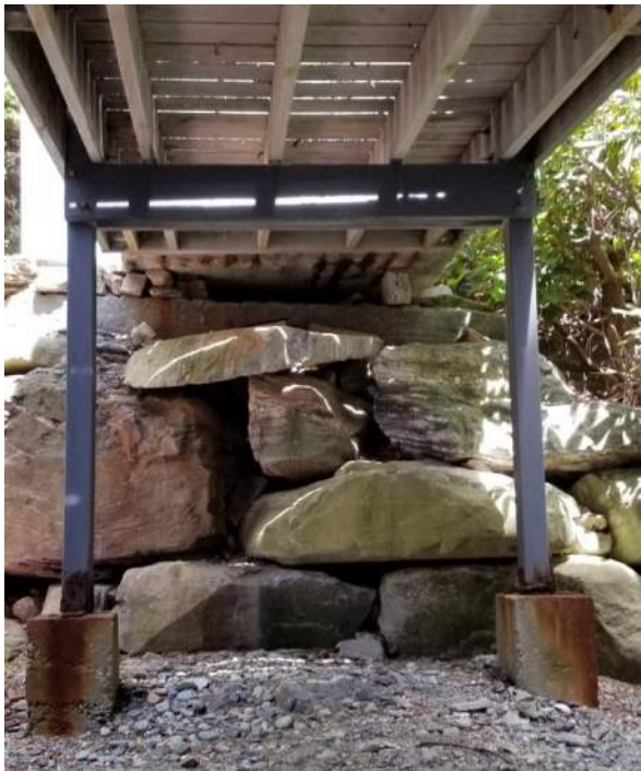
Photo S2: Rear entry ramp (underside view) and wood side stairway compromised.
