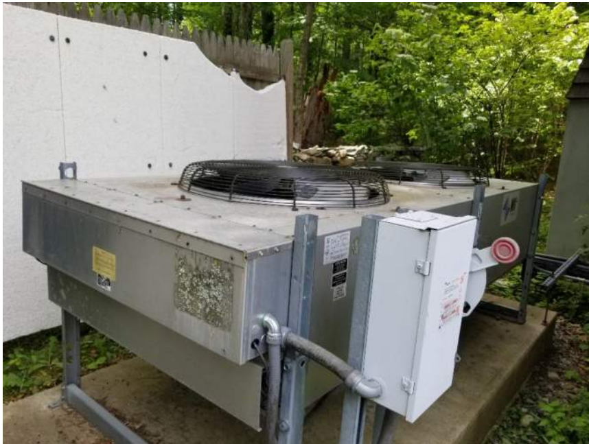
Photo H1: Condenser. Replace insulation and provide weather-proof UV resistant jacket.
