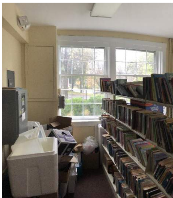
Photo E3,E4: Working space violation in front of panelboards. Remove stored items.
