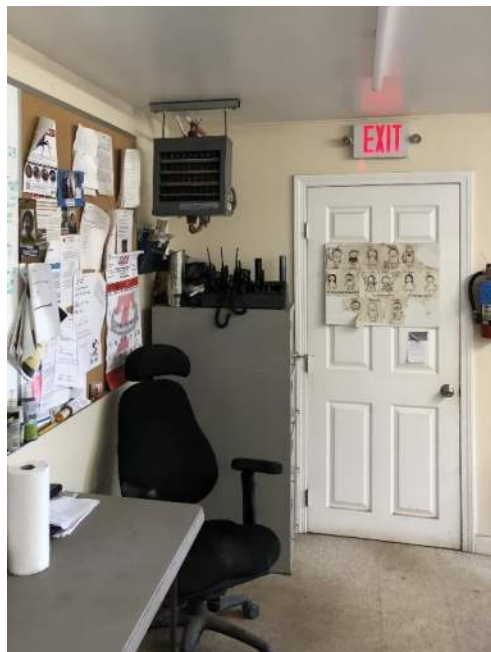
Photo E3: Install emergency lighting with battery backup (as shown in photo) where lacking throughout facility.
