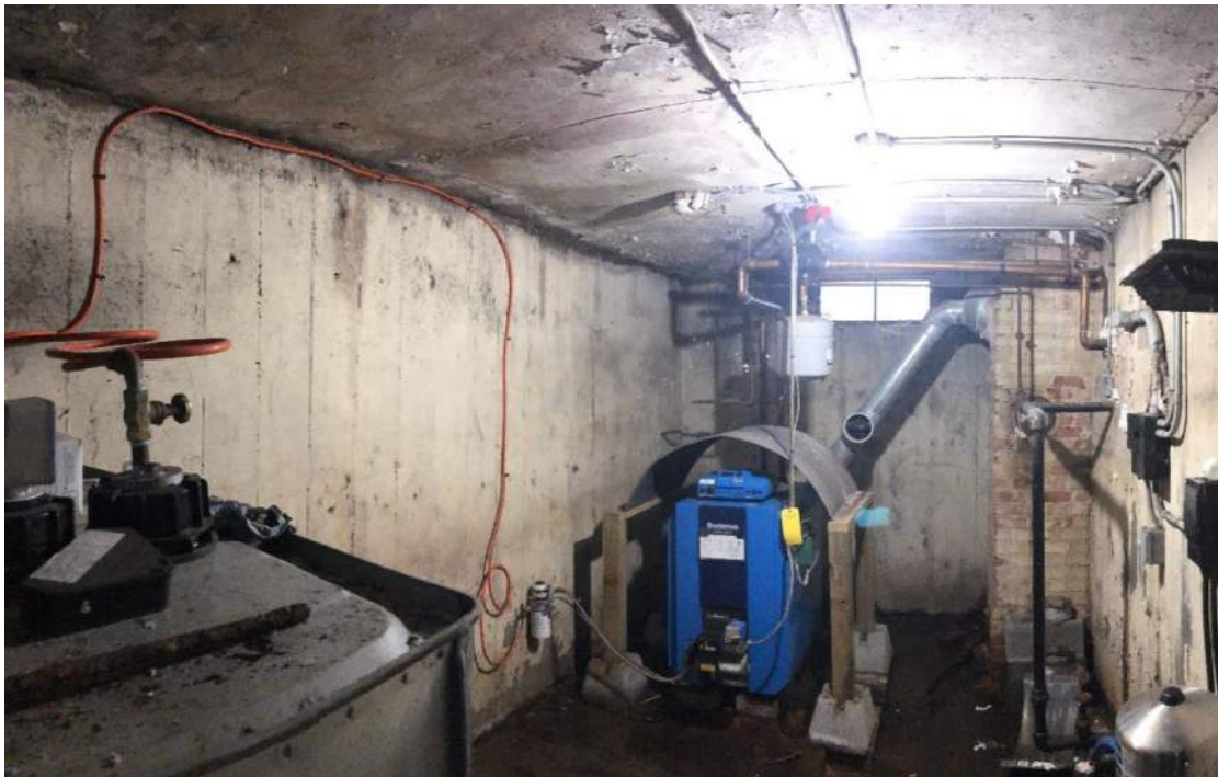
Photo H2: Boiler room subject to water inflow and resultant moisture issues. See Photo C1.
