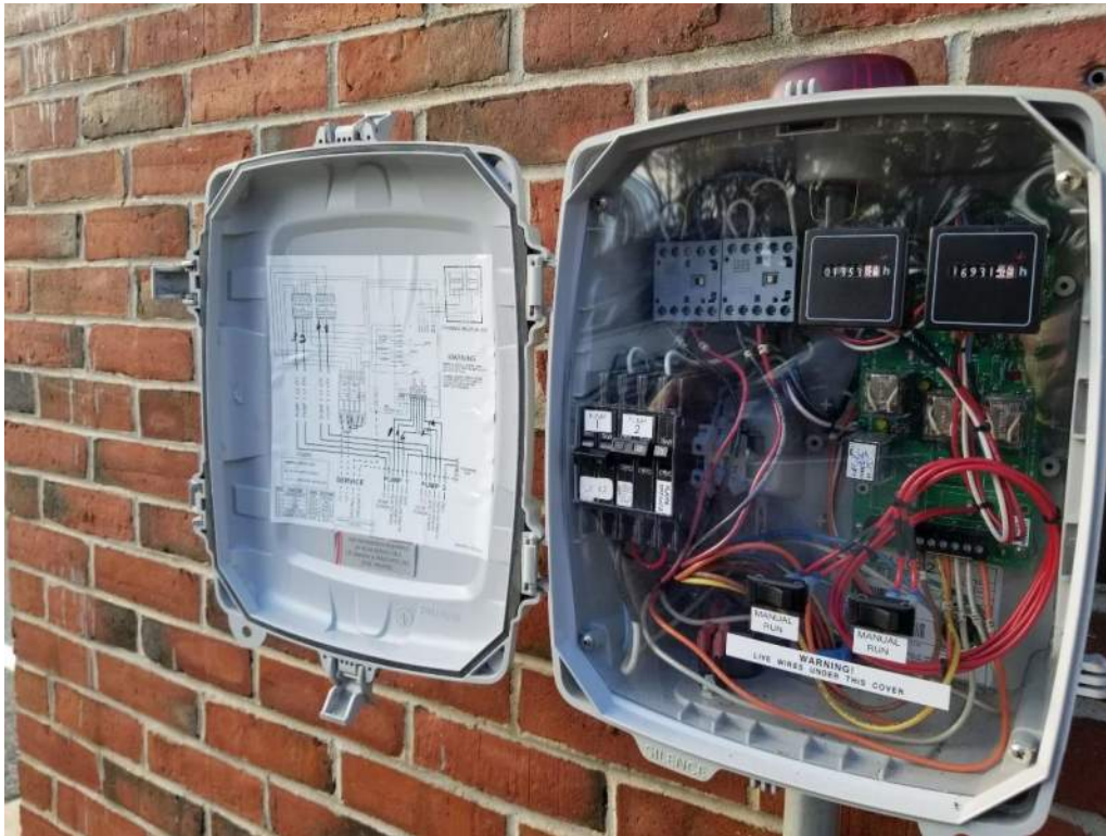
Photo C1: Photo of E-One Grinder Pump Control Panel. Power wiring and the control panel need replacement.
