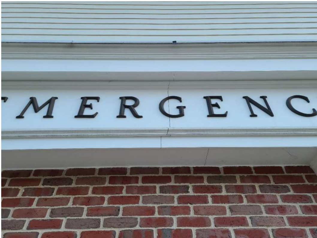
Photo S2: Trim joints to be caulked and repainted.
