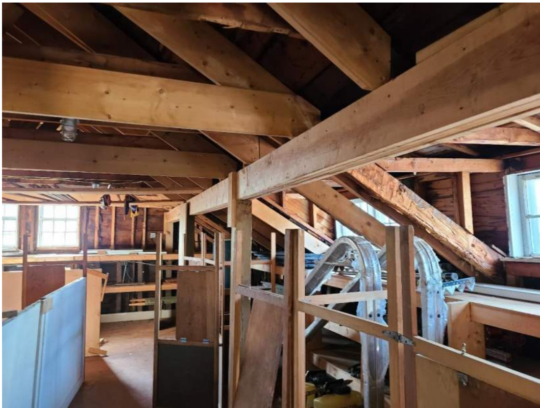
Photo S2: Supplemental header for roof rafters.
