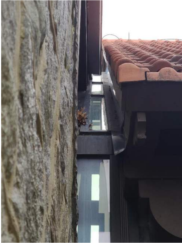
Photo S1: Expansion join between original building and addition is leaking.
