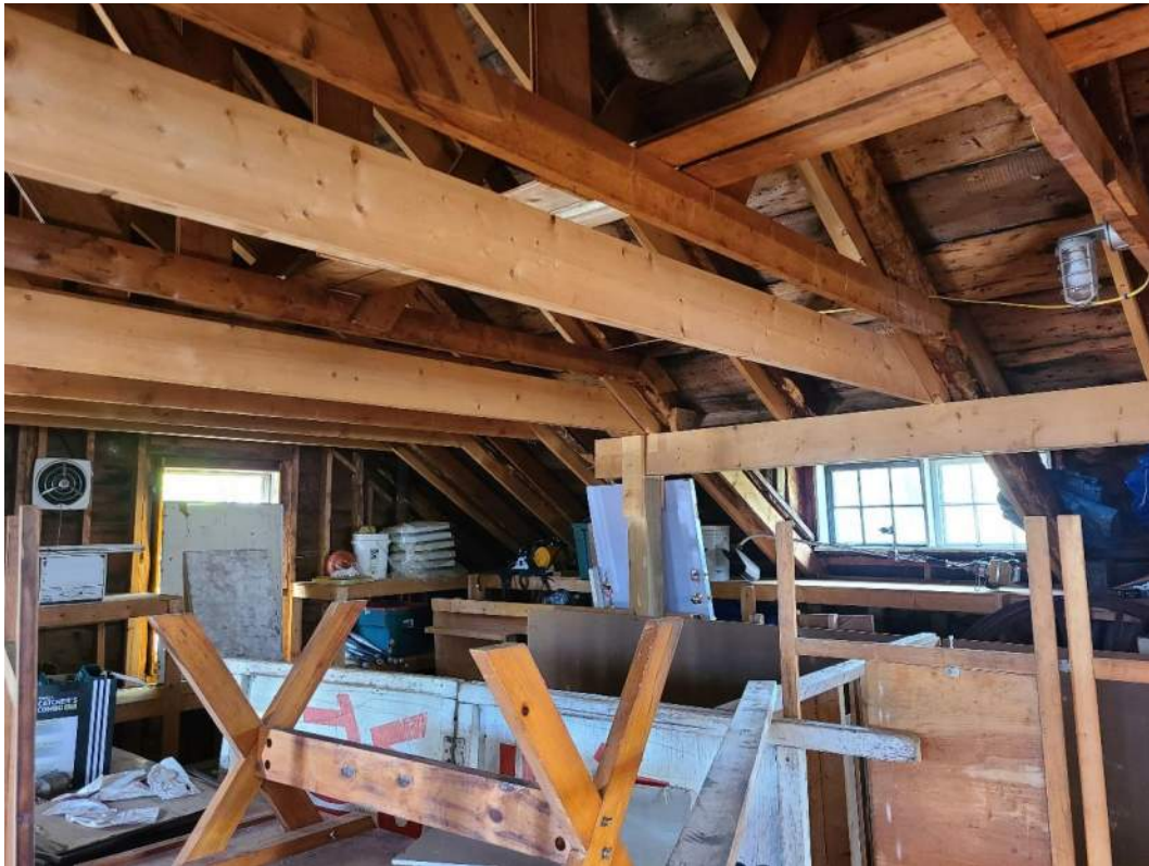
Photo S1: Patched and sistered structural framing in compromised old Fire Station.
