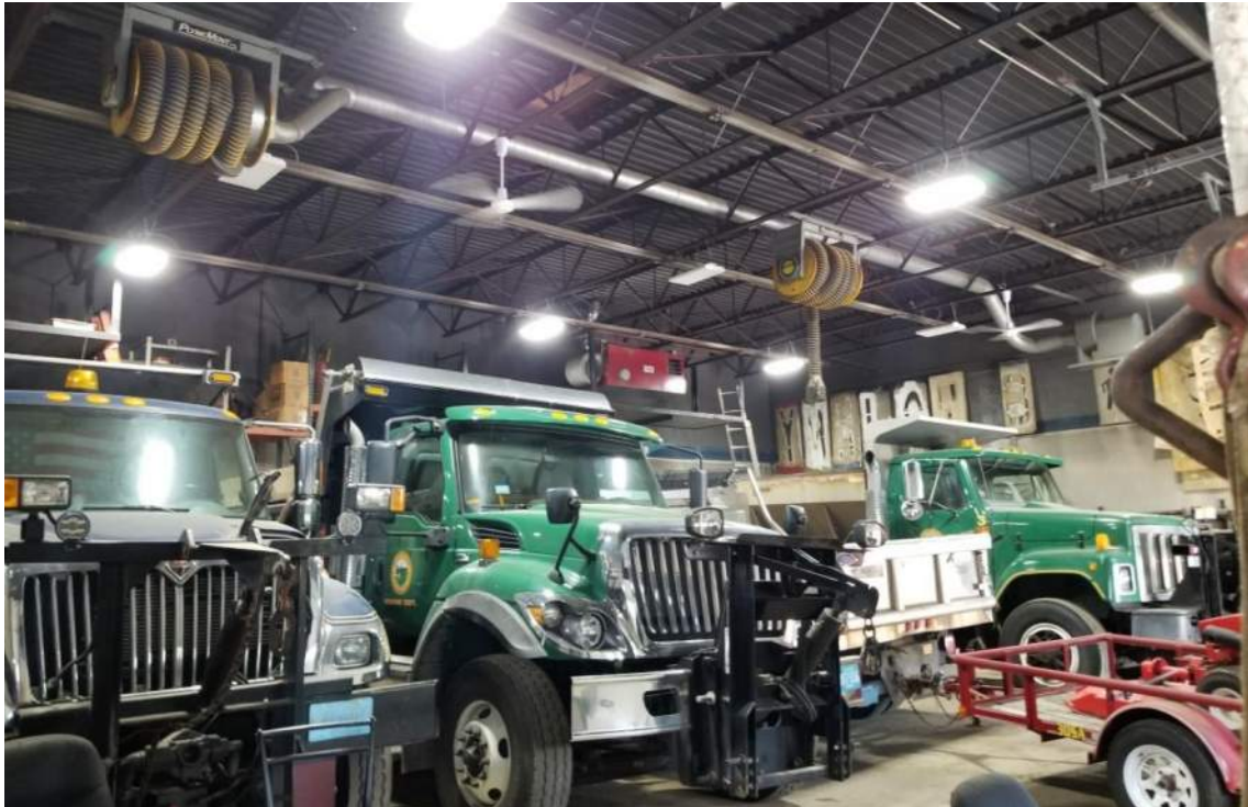
Photo H1: DPW Garage lacking automatic ventilation and gas detection is safety hazard. Need gray water tight tank, floor drains and an oil water separator. Lack of adequate spacing between vehicles for adequate operations and maintenance activities.
