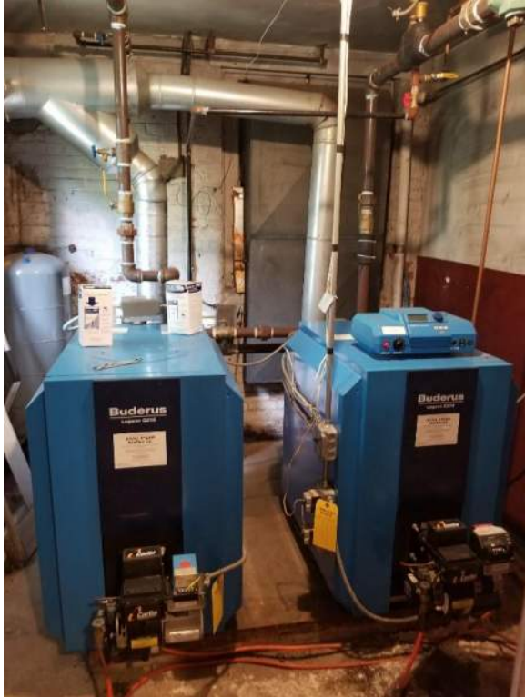
Photo H1/P1: Existing Boilers. Recommend water analysis and possible treatment to reduce hydronic system piping corrosion.
