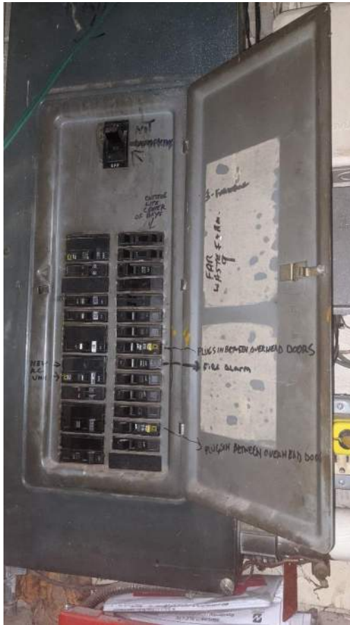
Photo E1,E2: View of the existing panelboard and ATS. Nearing end of useful life.
