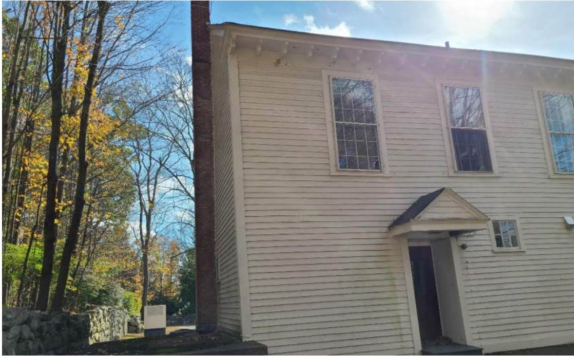
Photo S1: Eave and siding paint chipping.
