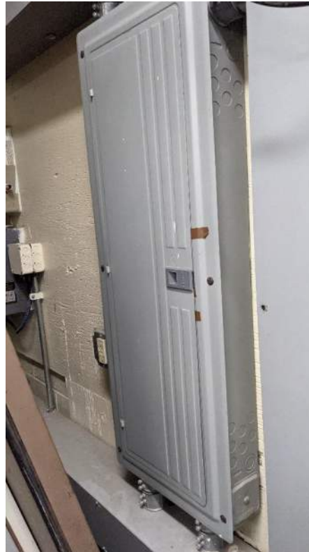
Photo E2,E3: Electrical panels. Ensure stored items cleared from front of panelboards to avoid working space code violation.
