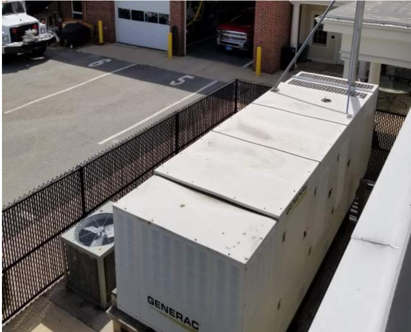
Photo E1: Backup generator is having mechanical issues and will likely require replacement in the next 5 years.
