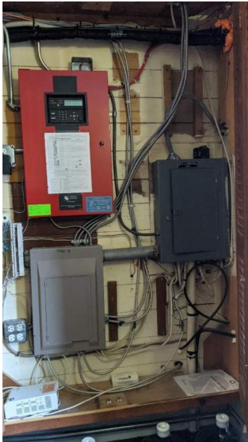
Photo E1,E2: View of the existing main distribution panel at end of useful life. Provide minimum 30-inch wide by 36-inch depth clear working space in front of electric panels.
