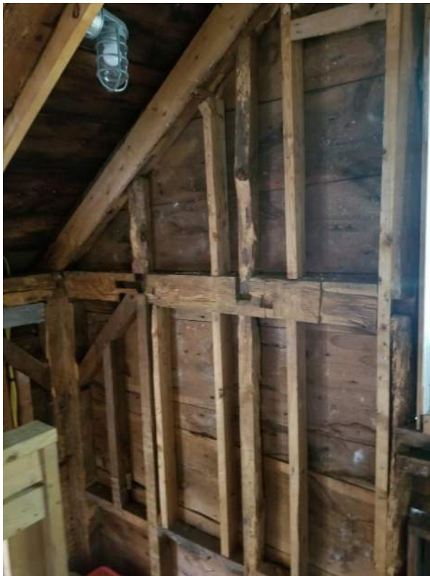
Photo S4: Original framing and siding in Old Fire Station second floor.
