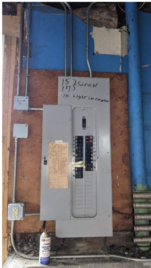
Photo E2: Electric panel. Install surge protection, code violation.
