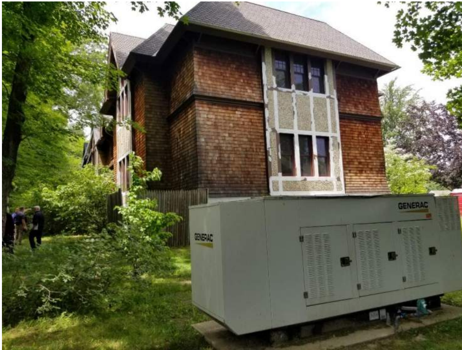
Photo E1: Backup generator. New motor recently installed after 10 years of operation.
