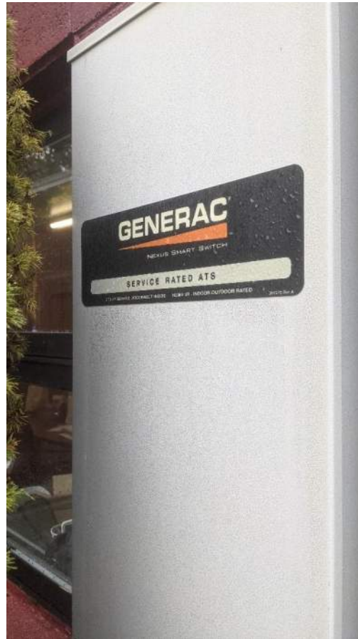
Photo E1,E2: View of the existing panelboard and ATS. Nearing end of useful life.
