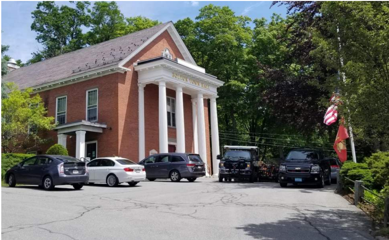
Photo C1: View of the front driveway. Guardrails compromised, need replacement. New curb required to prevent surface runoff down bank, behind retaining wall and onto street.
