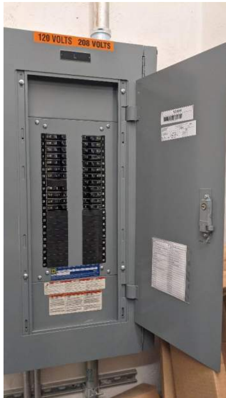
Photo E2,E3: Electrical panels. Ensure stored items cleared from front of panelboards to avoid working space code violation.
