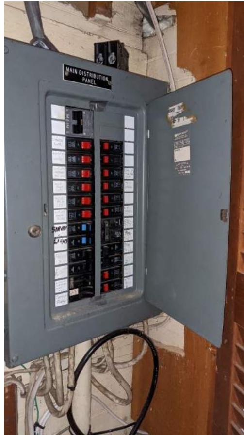
Photo E1,E2: View of the existing main distribution panel at end of useful life. Provide minimum 30-inch wide by 36-inch depth clear working space in front of electric panels.
