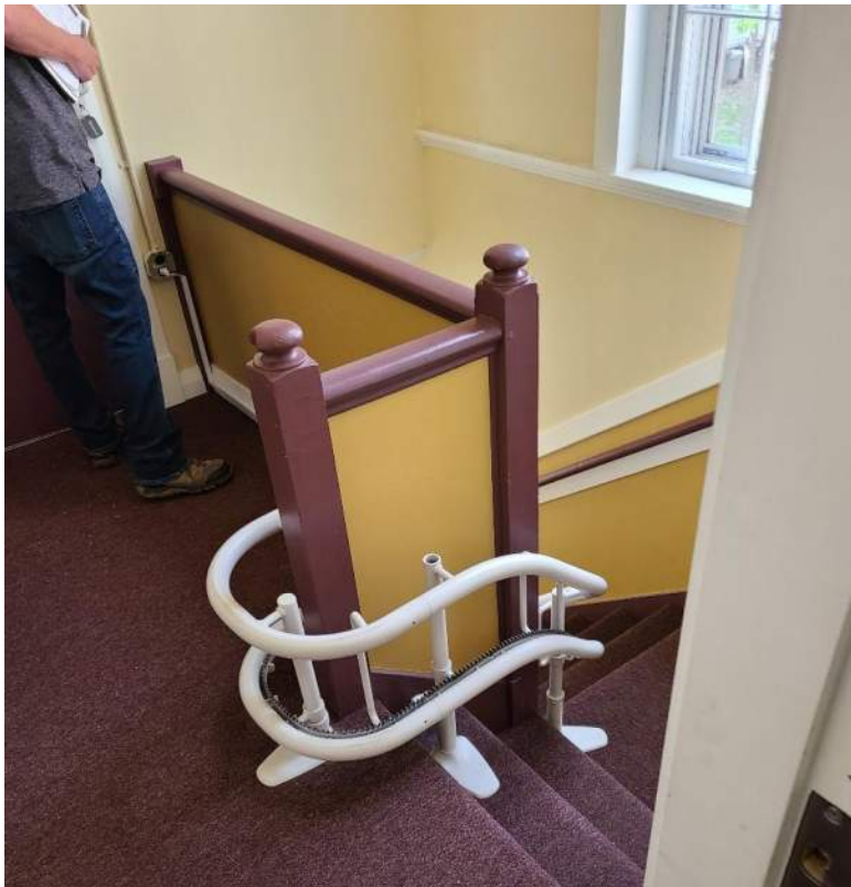
Photo S4: Half-wall is too low at top of stairs. Safety risk. Increase height.
