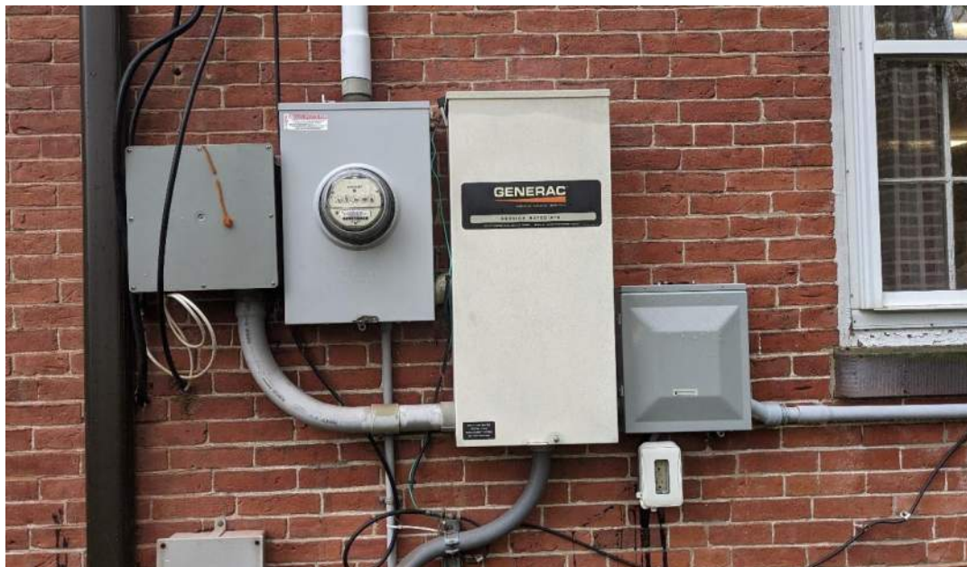
Photo E3: Automatic transfer switch and main feed.
