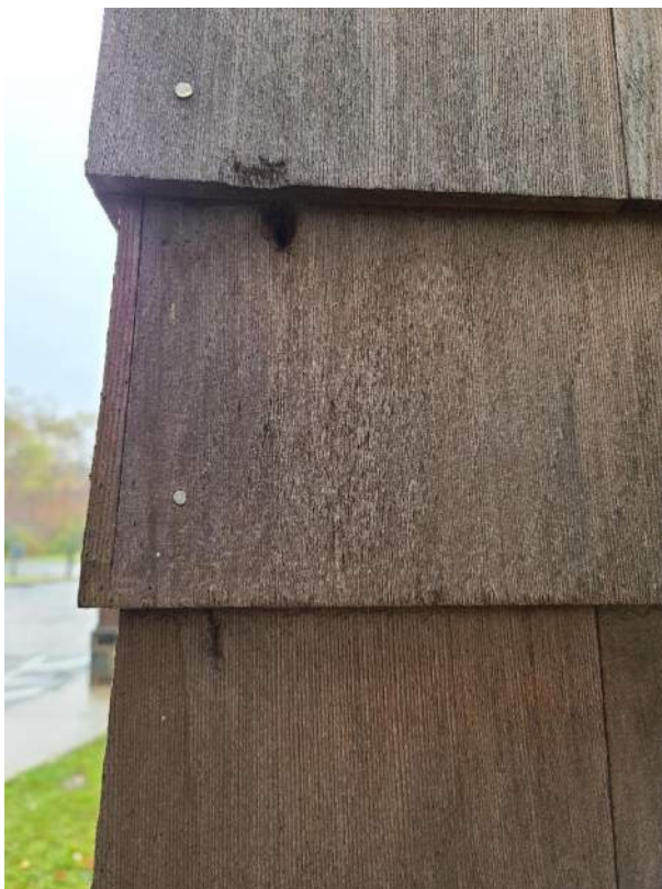
Photo S4: Holes in cedar siding from bugs or pests need to be sealed.
