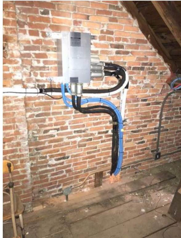
Photo H2,H3: There are air quality concerns in Town Hall; improved ventilation or air purification may be required. Photo of ductless mini-splits distribution box in attic.
