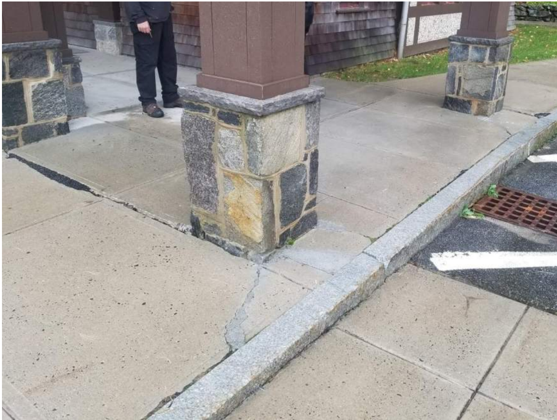
Photo C1: Sidewalk damage at main entrance. Granite curbing missing grout throughout.
