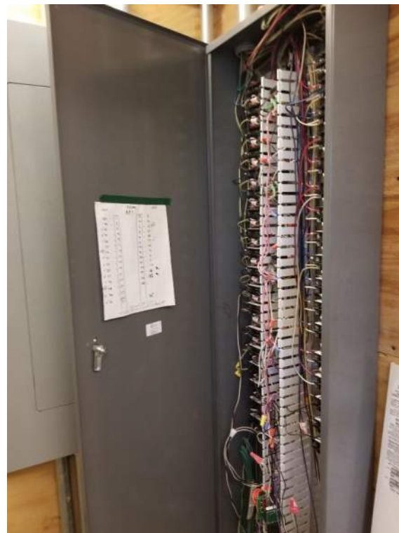
Photo E2,E3: Low voltage Payne Sparkman lighting control system is problematic. Electrical panels. System diagnosis by manufacturer required.
