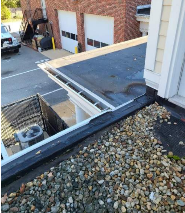
Photo S1: Guardrails needed on roof. Door too close to edge without fall protection.
