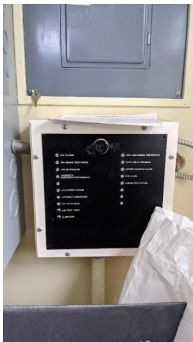
Photo E3,E4: Working space violation in front of panelboards. Remove stored items.
