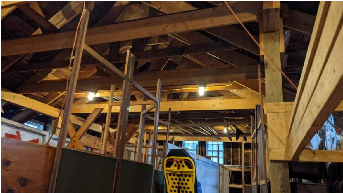
Photo E1: Second floor lighting. Building is lacking illuminated exit signs and emergency lightening, which are code violations.
