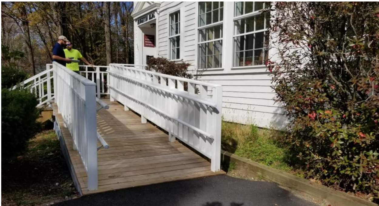
Photo C2: Entry ramp is not ADA compliant. Too steep ( >8.3\% ), no handrail extensions, lacks landing (60" level required).
