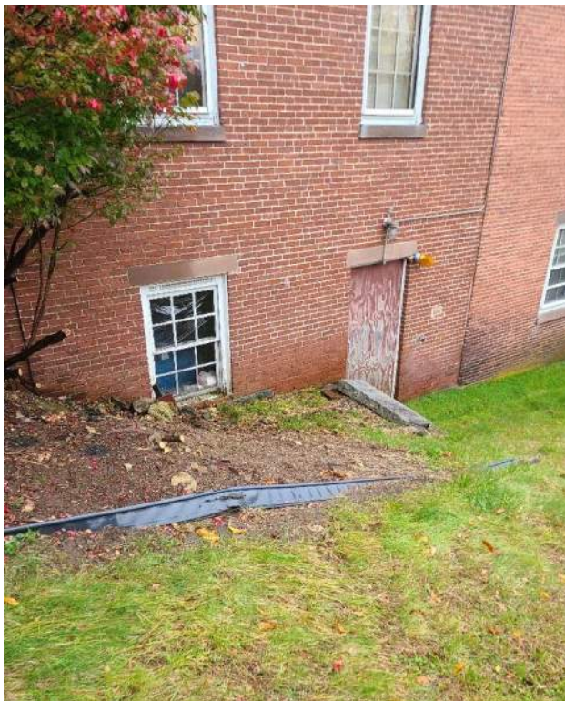
Photo C2: Surface runoff compromising SW corner of building. Regrade and install drainage.
