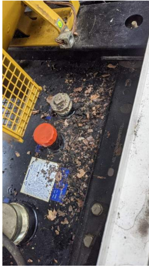
Photo E1,E2: Evidence of rodents in backup generator. Clean and make rodent-proof
