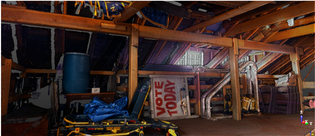
Figure 2 – Carrying beam along west side of roof framing
