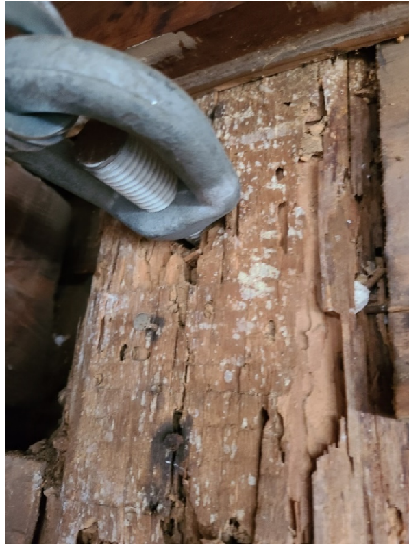
Photo 3 – Column B4 as observed after selective demo, extreme BID evident without removal of material.
