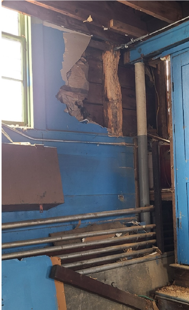
Photo 5 – Column A4 after scraping to remove surficial BID, note damage continues into member beyond loose material removal.
