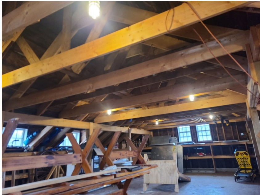
Photo 8 – Typical supplementary roof framing seen from second story floor. Note carrying beams background left and foreground right.
