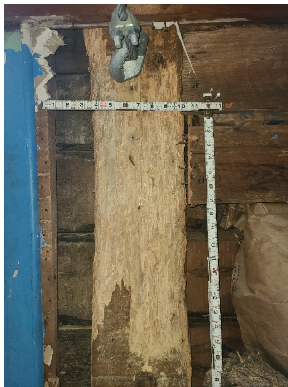
Photo 4 – Column A3 after scraping to remove surficial BID, note damage continues into member beyond loose material removal.
