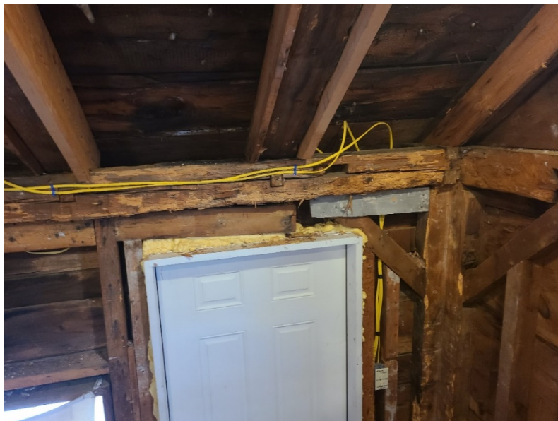
Photo 6 – Observed BID in top plate along Column Line A and in Corner Column A5
