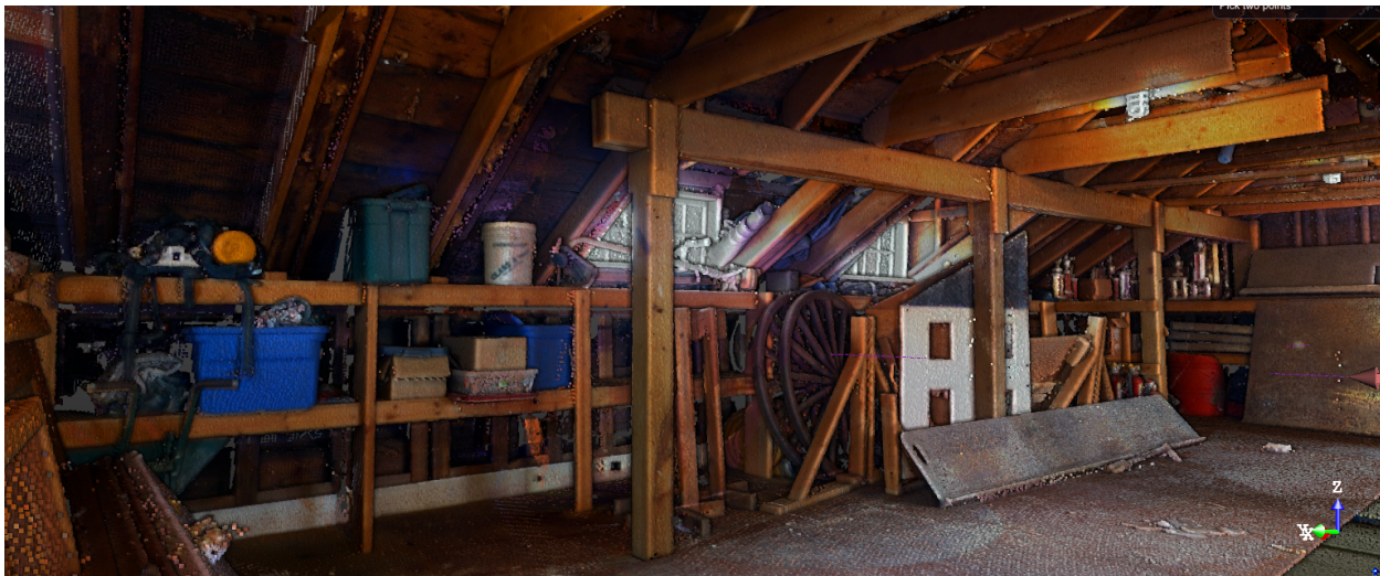
Figure 3 – Carrying beam along east side of roof framing.
