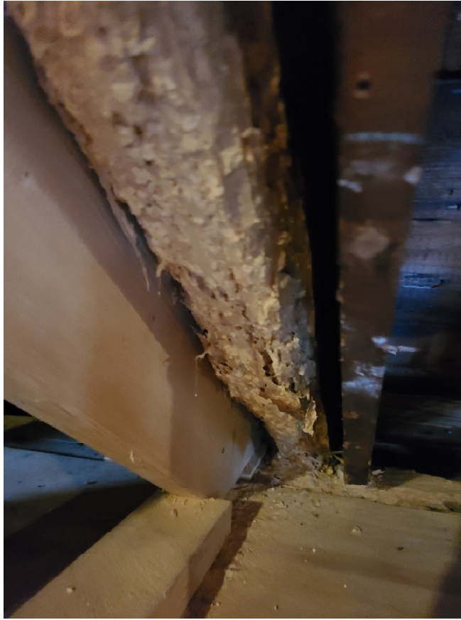
Photo 7 – Roof rafter with extreme BID along Column Line B Above Column B4
