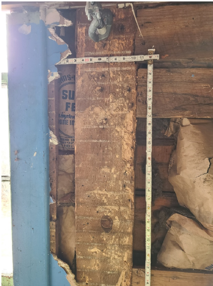
Photo 2 – Column A3 before, note evidence of BID on exterior of column
