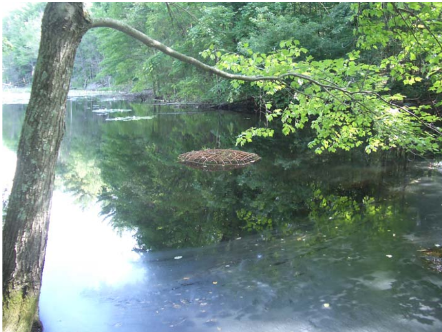
Photo #4: Screened inlet for spillway outlet pipe.
