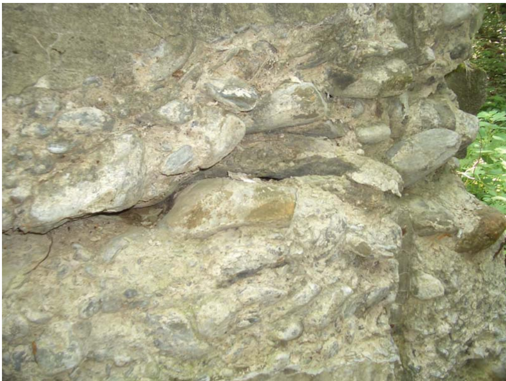
Photo #23: Major crack in the left spillwaywall downstream
