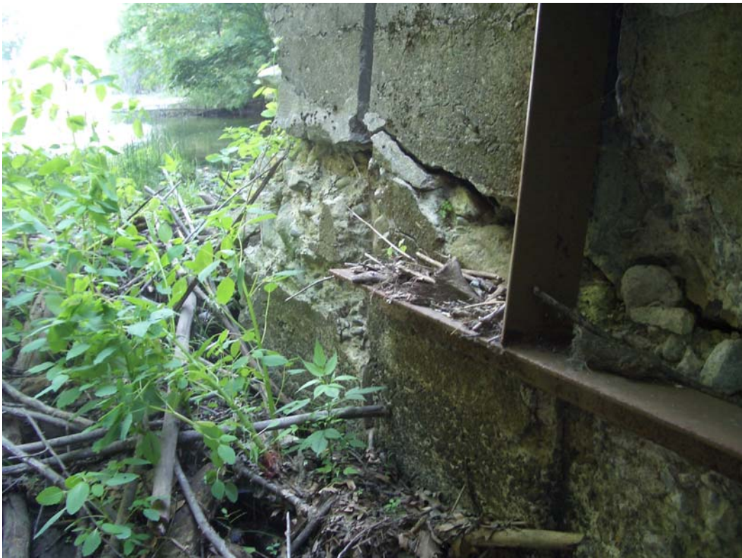
Photo #25: Major crack in left spillway wall ,upstream
