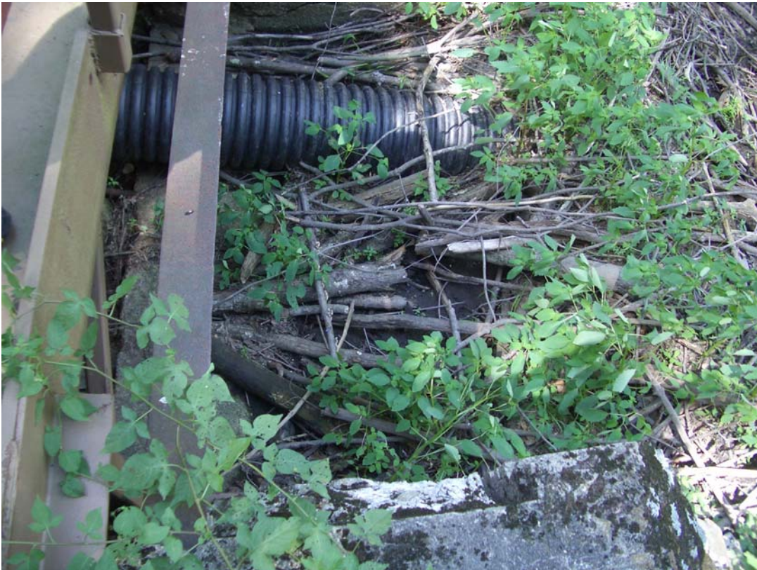
Photo #30: Debris dam at the spillway and pipe outlet.
