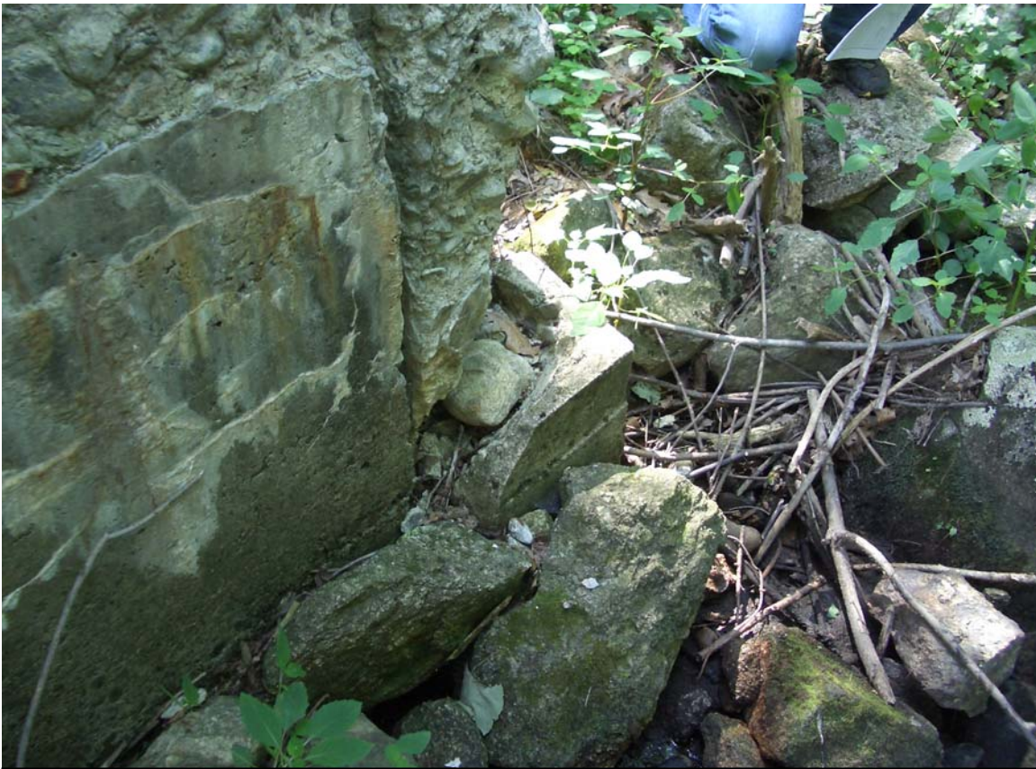
Photo #21: Deterioration of left, downstream spillway wall
