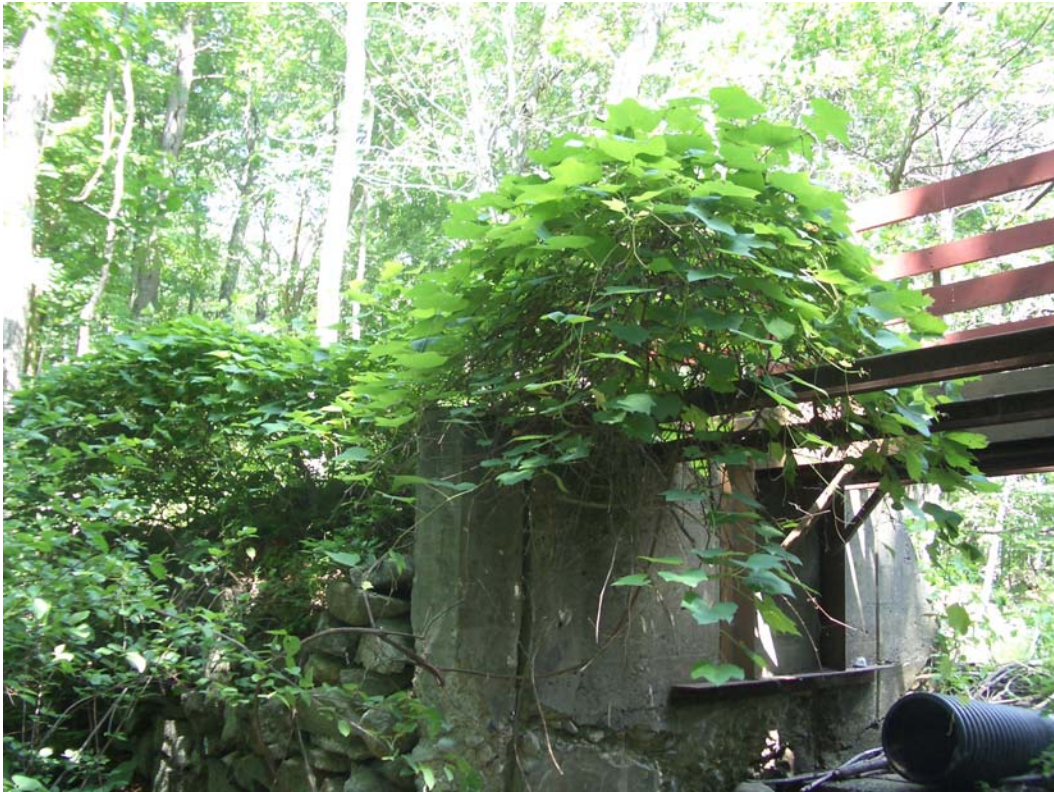
Photo #19: Downstream of spillway facing the right (west) spillway wall and dam wall with grape vine
