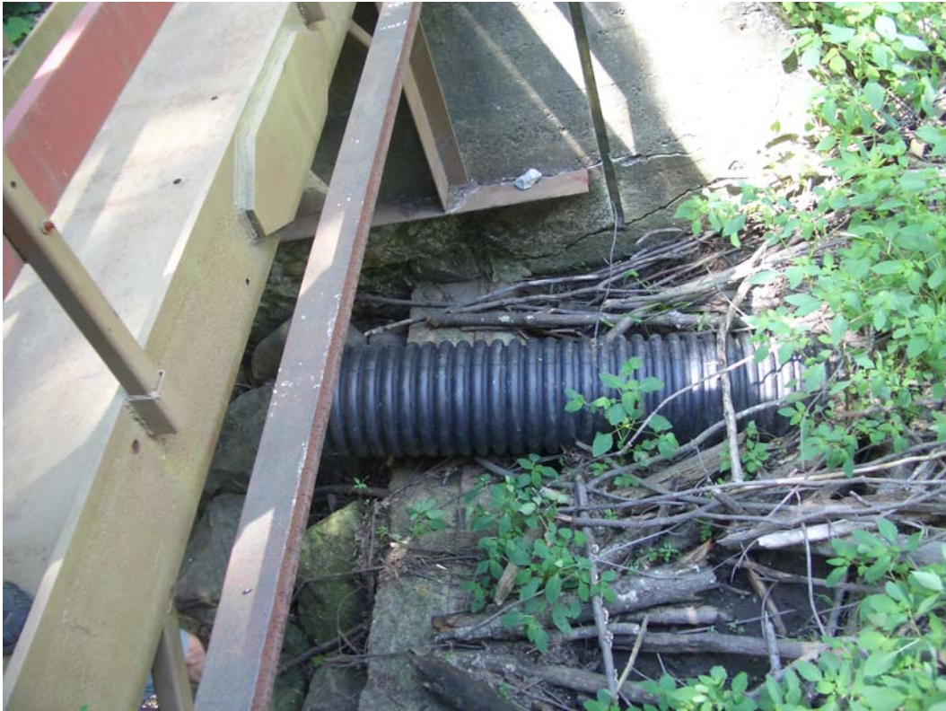
Photo #31: Debris dam at the spillway and pipe outlet.
