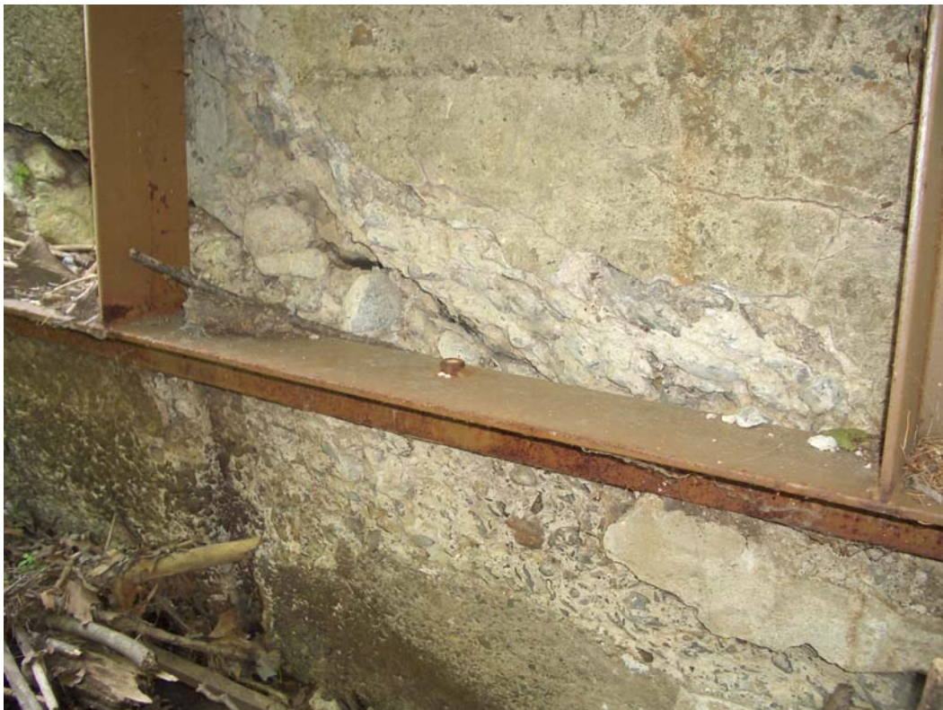
Photo #20: Major crack in left spillway wall and steel bracing
