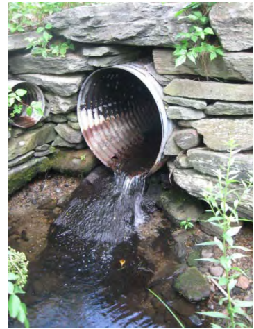
Figure 7: Perched culvert under Lancaster Rd.
