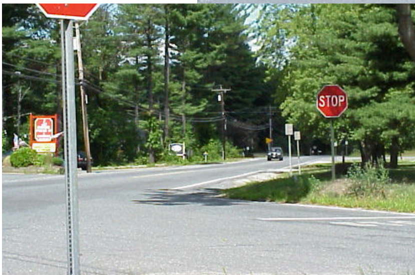
EXHIBIT 8 (Above) View west, exiting high school driveway onto Route 117. Sightline is inadequate for speed of oncoming traffic (45 mph). (Left) View west, exiting from Green Road; Sightline is improved.
