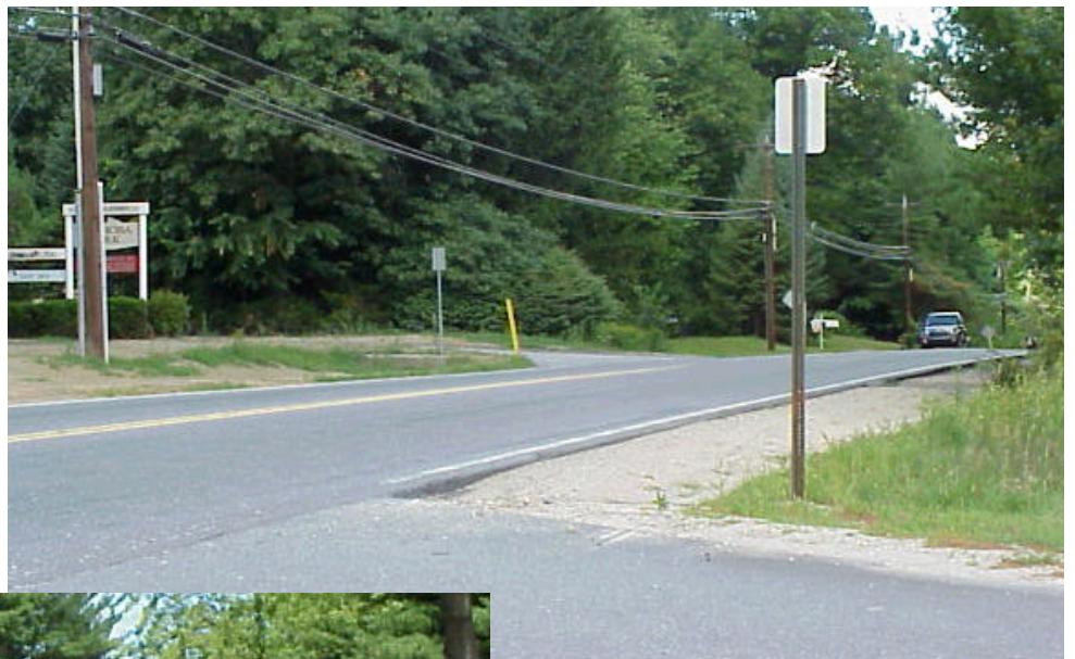
EXHIBIT 8 (Above) View west, exiting high school driveway onto Route 117. Sightline is inadequate for speed of oncoming traffic (45 mph). (Left) View west, exiting from Green Road; Sightline is improved.
