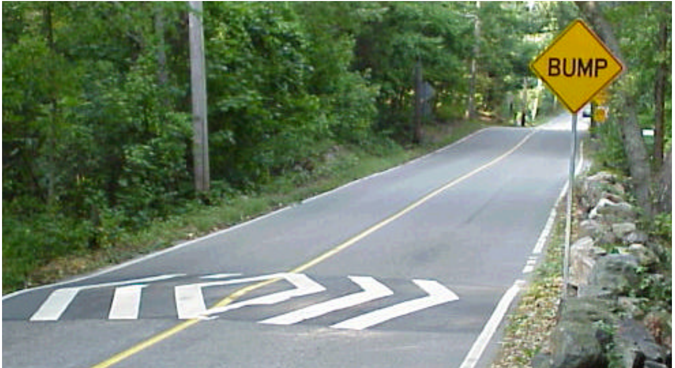
EXHIBIT 14 Speed bumps on Lexington Road, Weston, off Route 117. There are 5 speed bumps within a mile on this busy commuter shortcut. These wider bumps are well designed and extend to edge of roadway.
