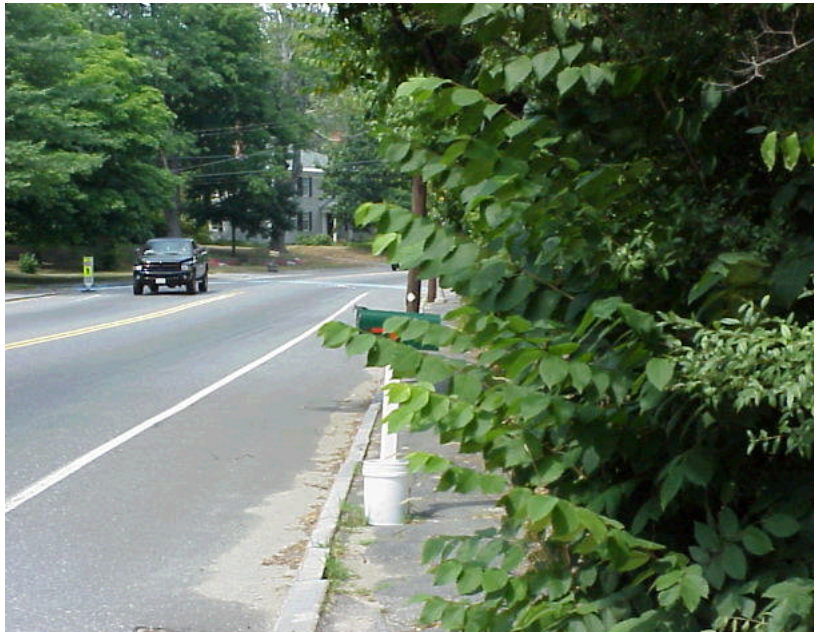
EXHIBIT 18 Sidewalk west of Federated Church driveway is impassable due to brush, sand, and uneven pavement.
